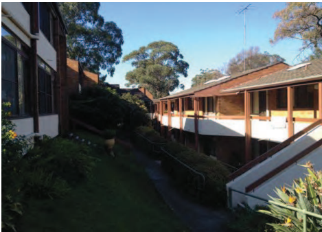
Embankments within site
