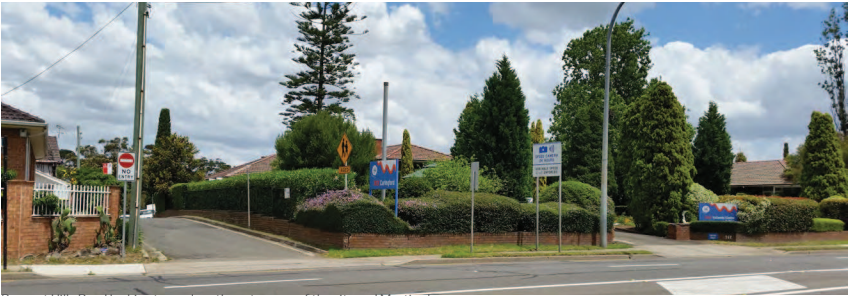
Pennant Hills Road looking toward north east corner of the site and Martins Lane
