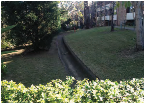
Existing storm water management device on site
